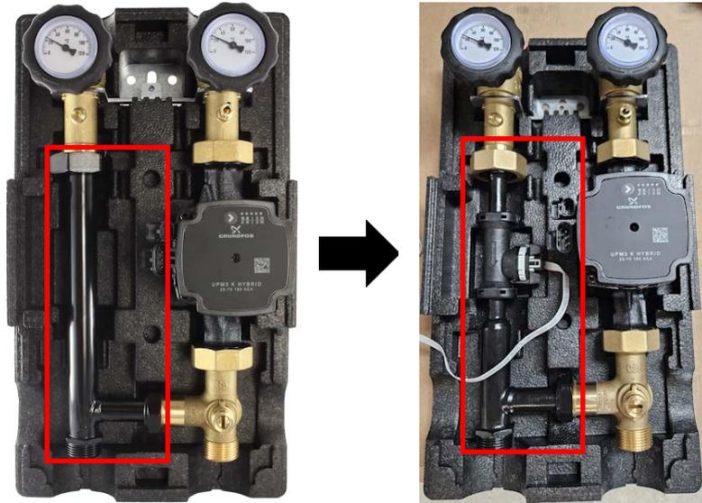
8. Put pipe insulation pieces back. Screw metal mount back on (ensure flow sensor cable remains accessible to controller).
