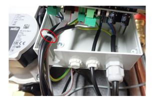
3. Unplug old valve from the electronics board.
